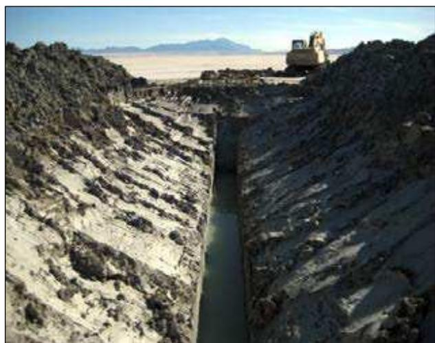
The lake brine shall be collected in a trench (as at right) or from extraction wells and pumped into a series of three solar evaporation ponds. Water shall be evaporated from the brine and salts would be selectively precipitated onto pond floors. The potash salts would be
