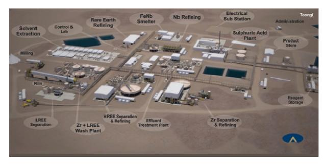
Sulphuric acid used for leaching will be produced on site using a sulphur burning acid plant that also generates electricity and steam for the process plant. A small amount of waste rock will be extracted and transported to a small waste rock emplacement to the southwest of the open cut. The liquid and solid residues from the processing plant will be transported and stored in liquid residue storage facilities, solid residue storage facilities and salt encapsulation cells.
