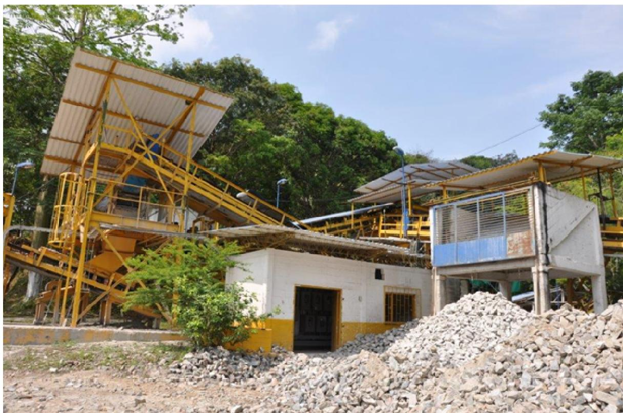
The crushing plant (pictured above) historically operated one shift per day at 10-12 tonnes per hour but has capacity of 20 tonnes per hour, providing sufficient crushed rock to feed the mill. The crushing plant consists of a jaw crusher, cone crusher, vibrating screen and associated belts and bins. A nominal 3/4" product is supplied to the mill.
